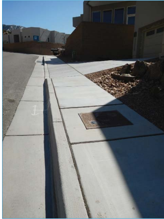
Typical concrete walkway
